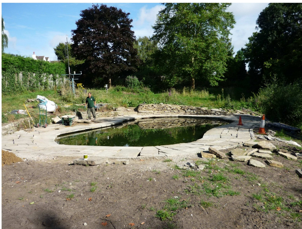
Figure 1: New pond under construction at Kenwood Nursery Yard as part of CBT project
